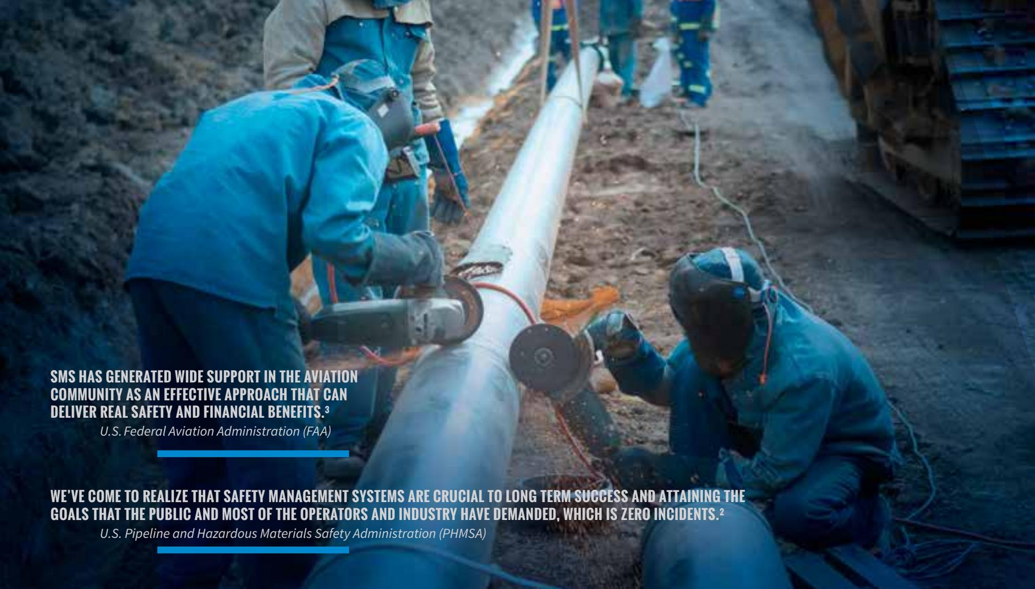
A photograph showing several workers in blue protective suits and hoods working on a large white pipe. They are using angle grinders to cut or grind the pipe. The scene is outdoors, possibly at a construction or maintenance site. The workers are focused on their task, and the overall atmosphere is one of industrial safety.
